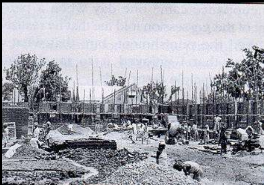
Construction of Loyola School
